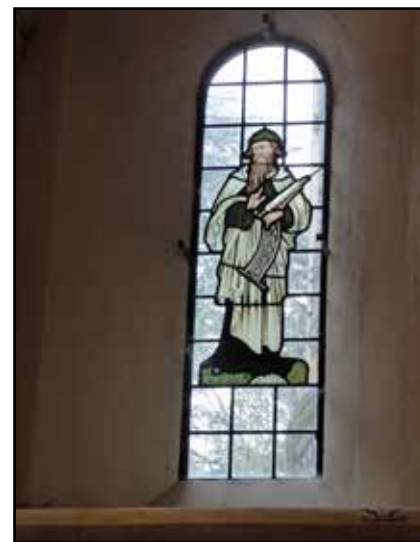
One of the original lancet windows. Note the thickness of the wall. The stained glass is a Victorian addition.
