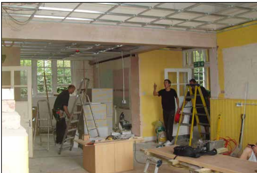
Figure 18 Showing new steel beam in place
