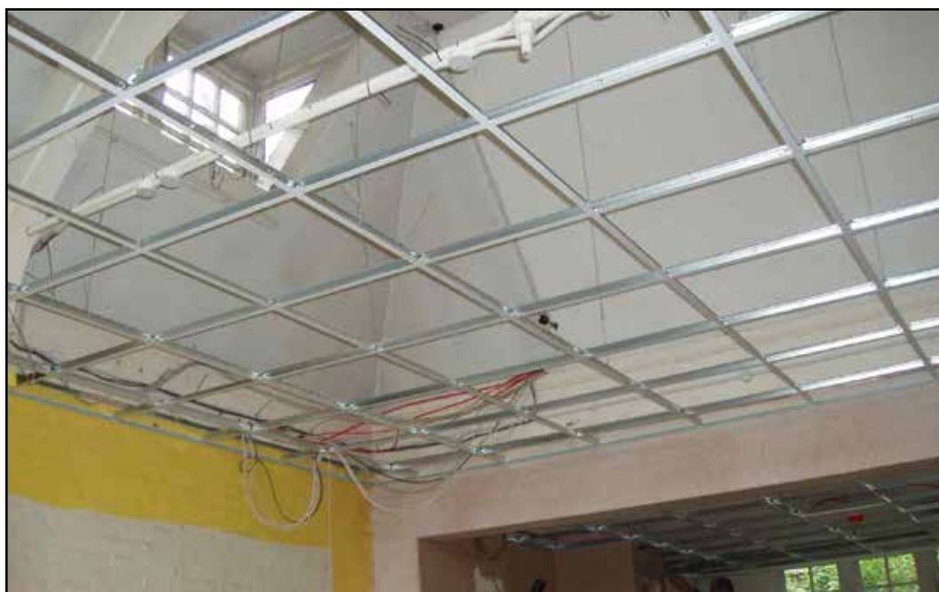
Figure 19 Construction of false ceiling
