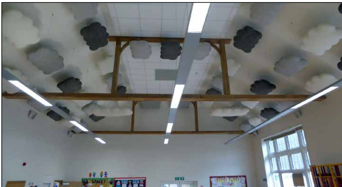
In 2019 the Friends of the School raised the money for and installed acoustic 'sound clouds' in the School Hall. These have been very successful in reducing noise and reverberation.
